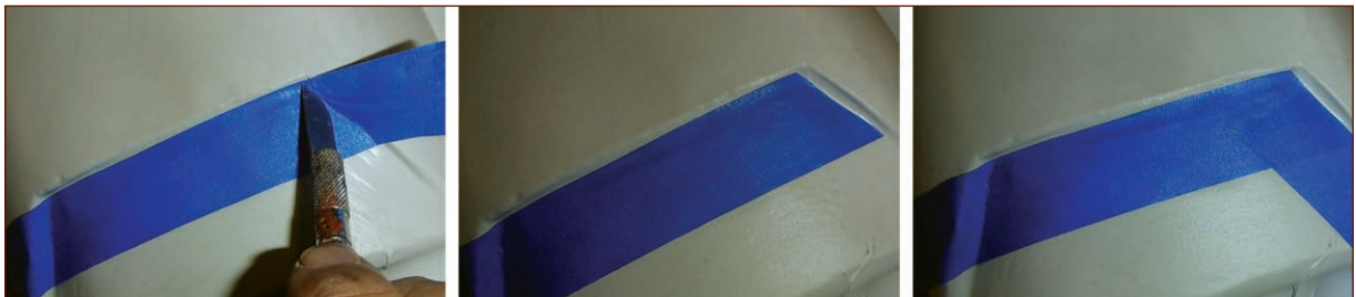
FIGURE 11-21: Cutting the tape after placing it against the corner makes for a nice, sharp corner.
