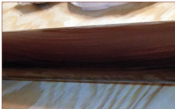
FIGURE 12-14: Visible brush strokes do a good job of simulating tight-knit wood grain similar to hardwood.
