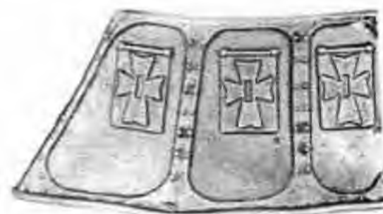
STEAM TANK LEFT SIDE ARMOUR 020204202
